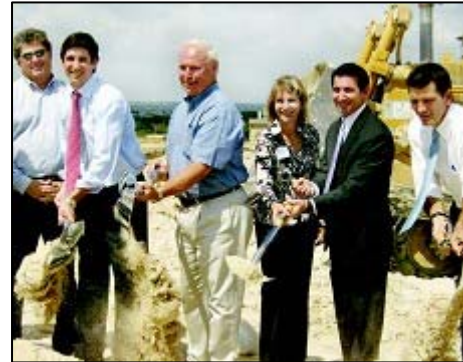
Civic leaders and staff from Simpson Vedder & Company and Kirksey Architecture Thursday break ground for the 257,000-square-foot Frontera Vista office building.
